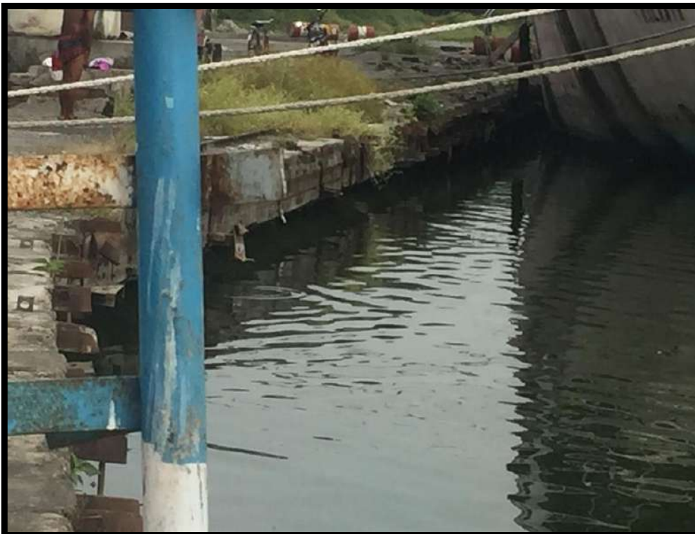
BERTHING FACE JUNCTION OF BERTHS 2 AND 4
