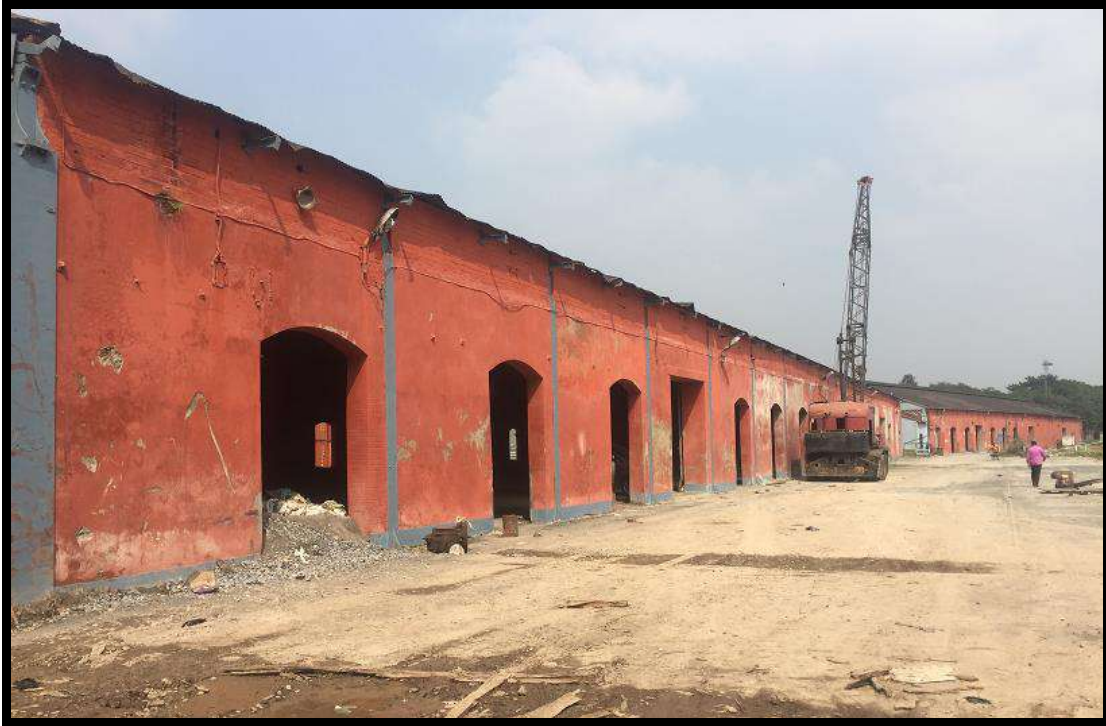
FRONT VIEW OF SHEDS Nos 2 & 4
