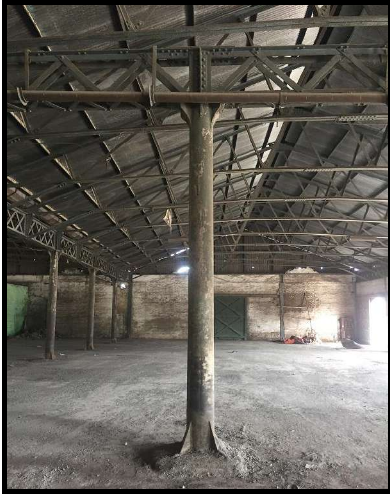
STEEL COLUMN SUPPORTING THE LATTICE GIRDER
