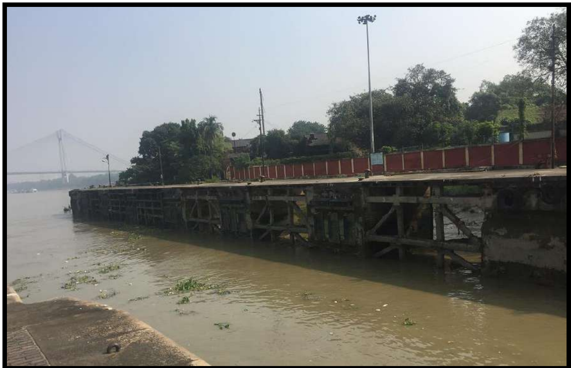
LEAD-IN JETTY FOR ENTERING KIDDERPORE DOCKS
