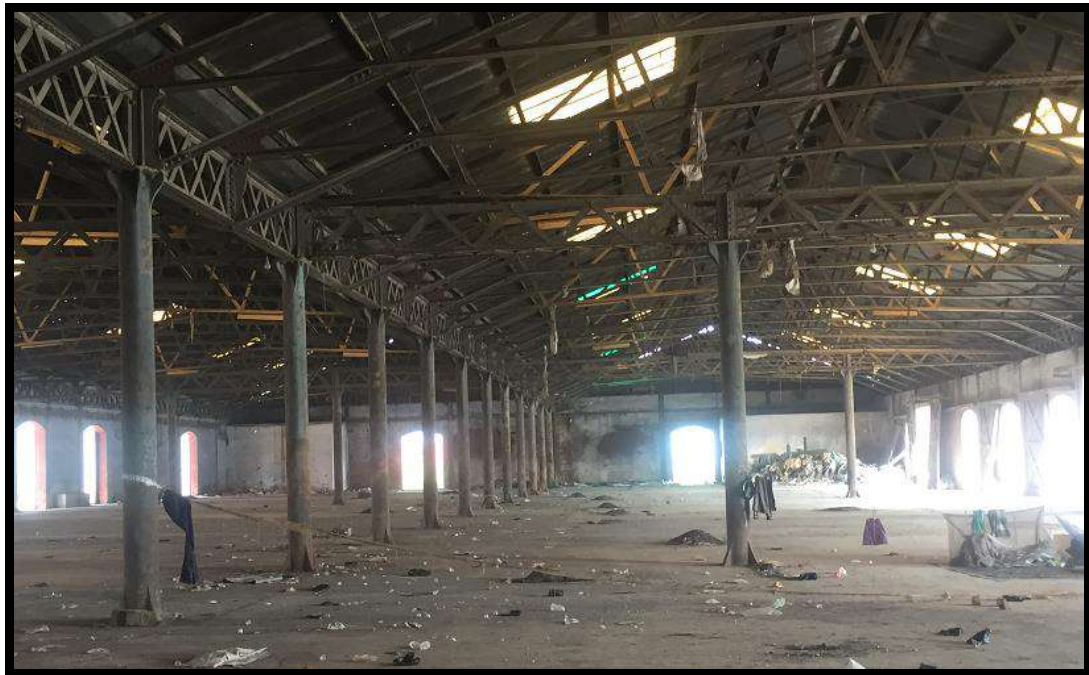
ONE MORE VIEW OF SHED INSIDE
