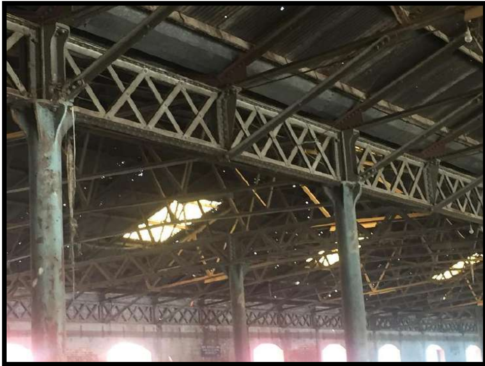
STEEL COLUMN SUPPORTING THE LATTICE GIRDER
