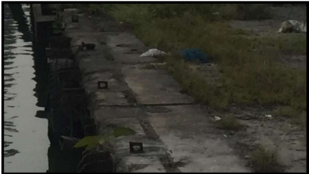
SURFACE OF BERTH No.4
