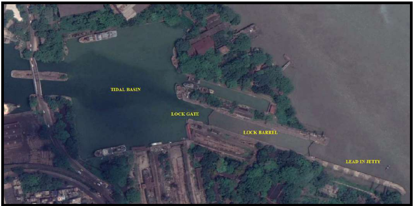
KIDDERPORE DOCKS – LOCK GATE AND TIDAL BASIN
