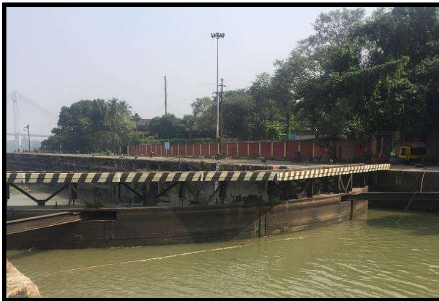
INSIDE VIEW OF THE LOCK GATE
