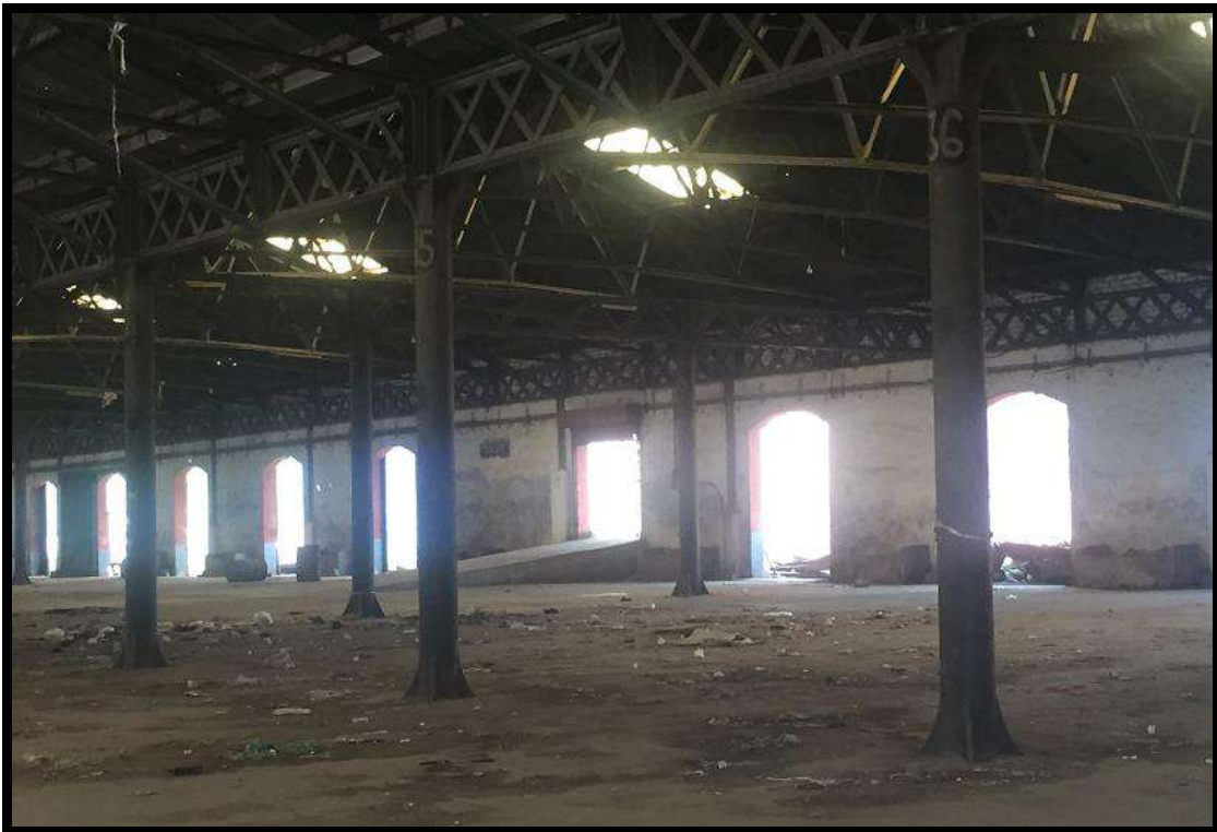
INSIDE VIEW OF THE SHED
