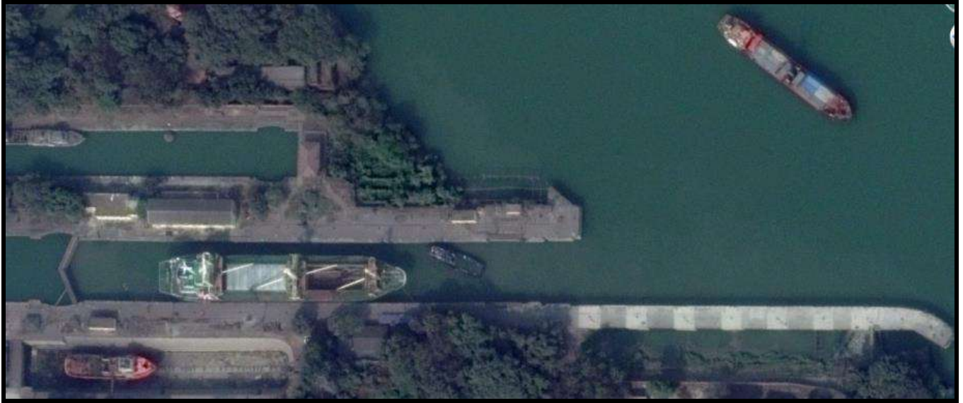
A VESSEL INSIDE THE LOCK BARREL
