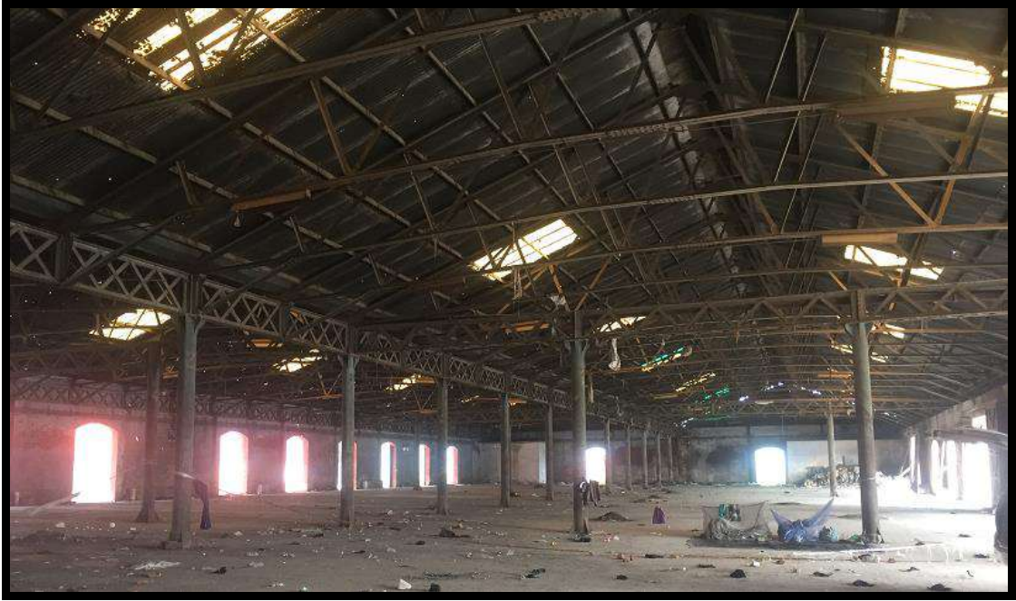
ANOTHER VIEW OF SHED INSIDE
