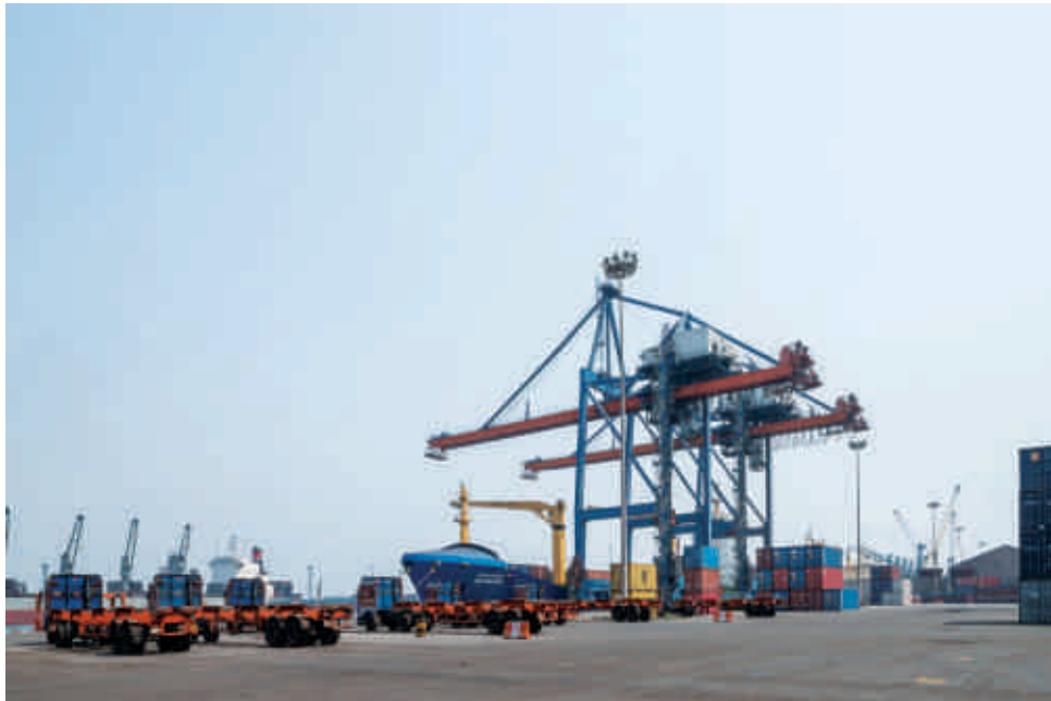
“RMQC operation at Container Terminal at HDC”
