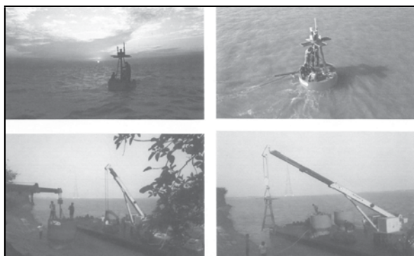
Fabrication, installation and deployment of ATGs
