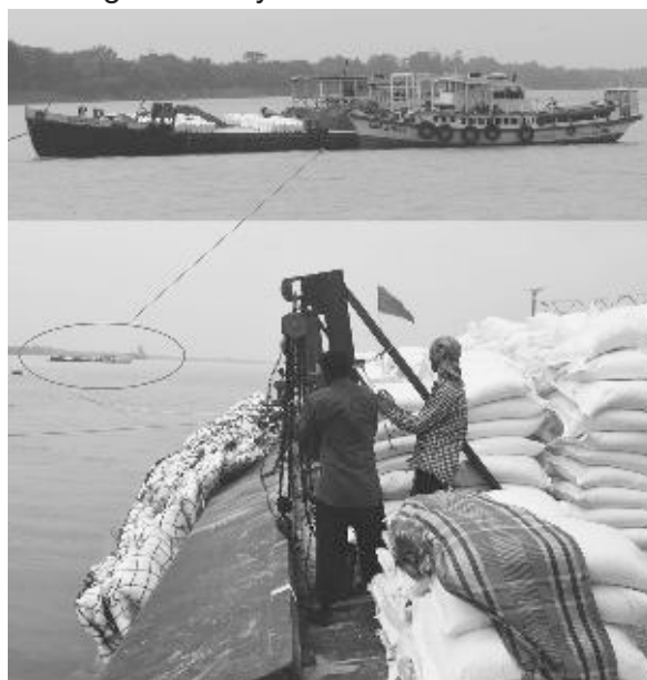
Ongoing execution of nourishment of Spur No. 92-A at Moyapur
