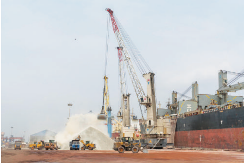
“Clean cargo being unloaded by MHC at Berth No. 13 at HDC”
