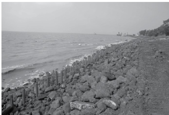
Bank protection works at Haldia
