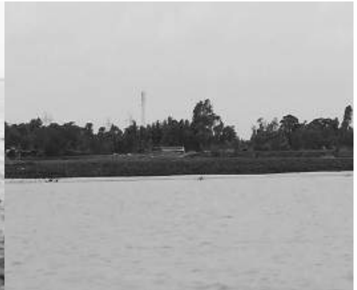
Bank Protection (Phase-I) at Shalukkhali
