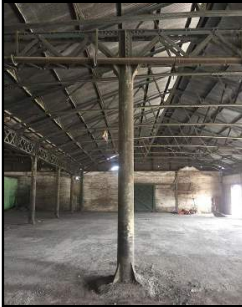
STEEL COLUMN SUPPORTING THE LATTICE GIRDER
