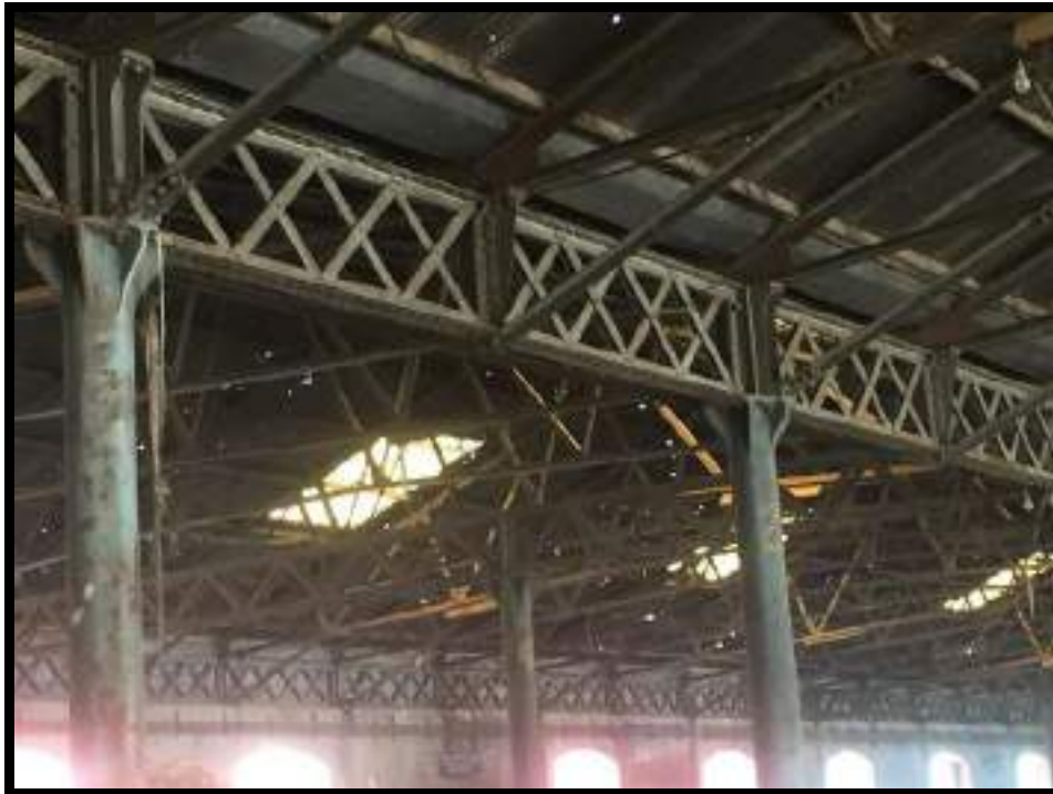
STEEL COLUMN SUPPORTING THE LATTICE GIRDER
