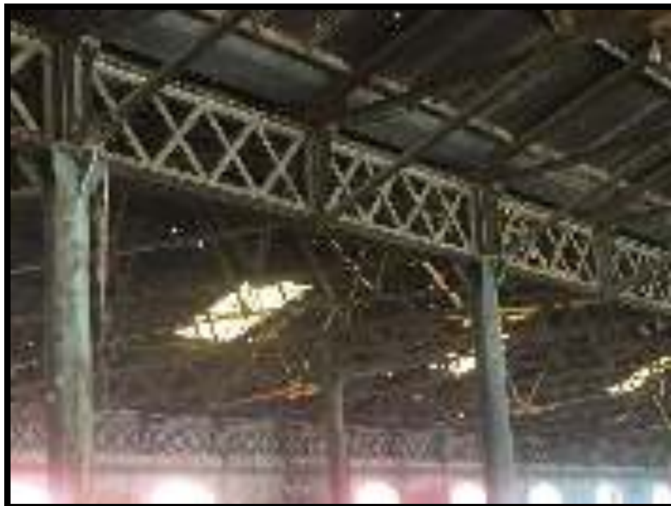
STEEL COLUMN SUPPORTING THE LATTICE GIRDER
