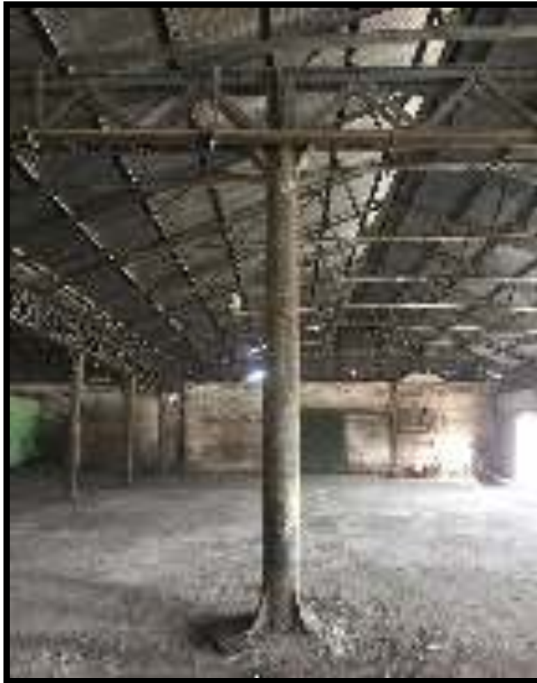
STEEL COLUMN SUPPORTING THE LATTICE GIRDER
