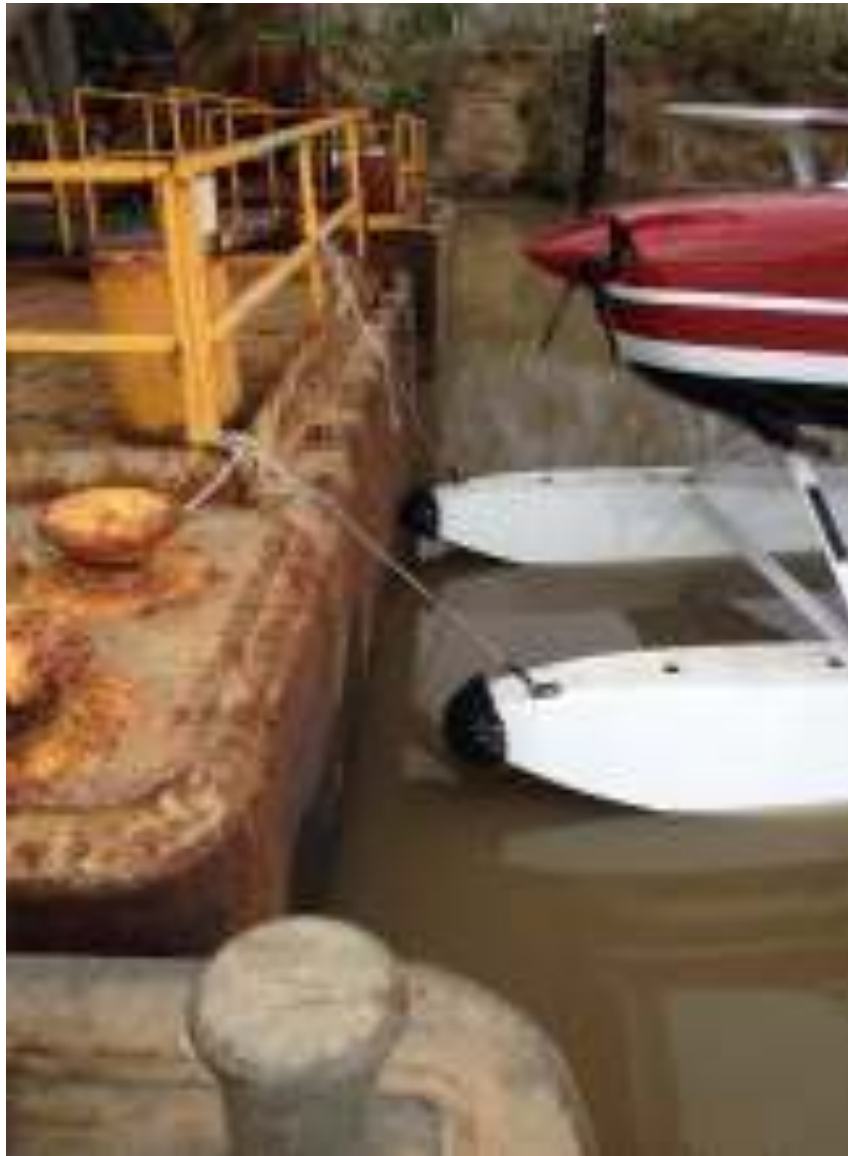
FIGURE 17 EXAMPLE OF FIXED DOCK WITH PARKING RAMPS
