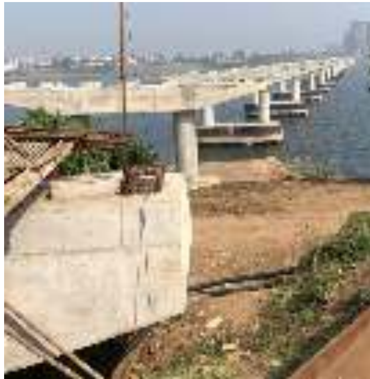
FIGURE 26 UNDER CONSTRUCTION BRIDGE NEAR AOI
