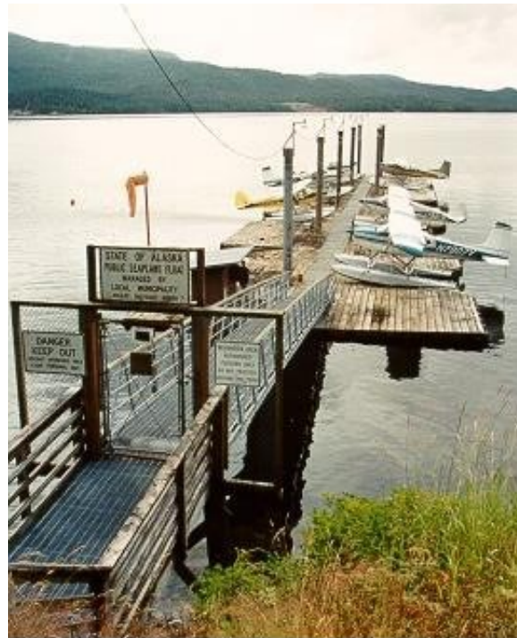
Figure 12 Example of a Gangway
