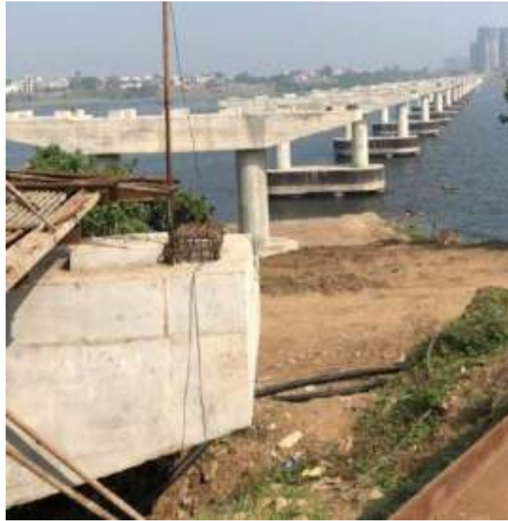
FIGURE 26 UNDER CONSTRUCTION BRIDGE NEAR AOI
