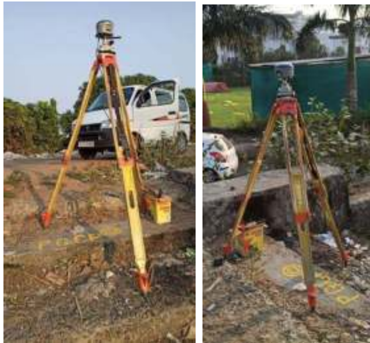
FIGURE 28 ESTABLISHMENT OF PRIMARY GROUND CONTROL POINT
