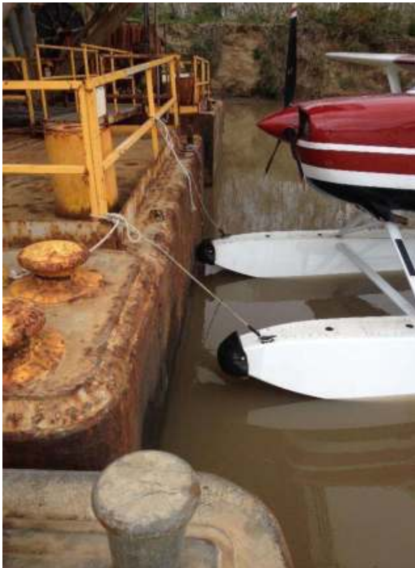
Figure 15 Example of Fixed Dock with Parking Ramps
