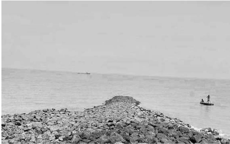
A spur at Nischintapur, nearing completion of nourishment work
