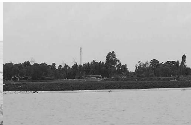
Bank Protection (Phase-I) at Shalukkhali
